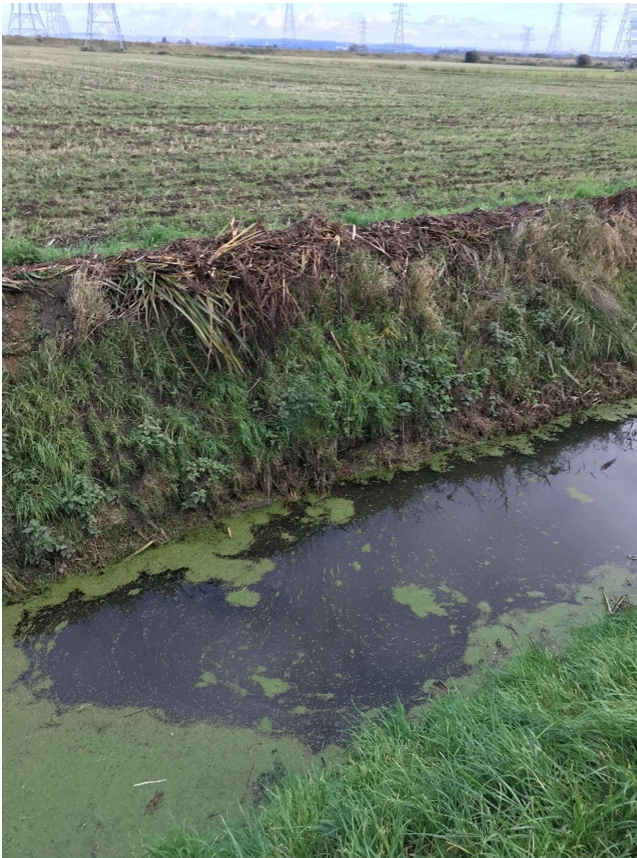
Photograph 11 – Keadby Common Drain adjacent to Chapel Lane, Keadby
